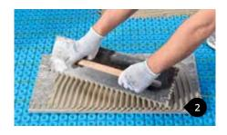
Apply the mortar to the back of the tiles with a notched trowel and lay them on the layer of mortar previously applied. Occasionally remove and check some tiles, to ensure full back coverage.
